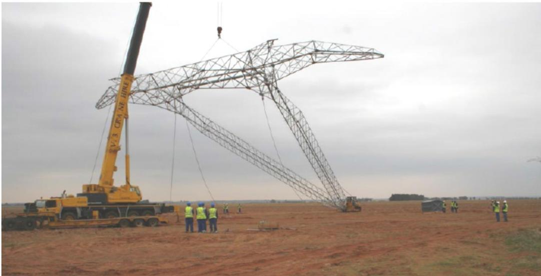
**Figure 10. During construction of new infrastructure (Gyed V-pylons)<sup>10</sup>**
